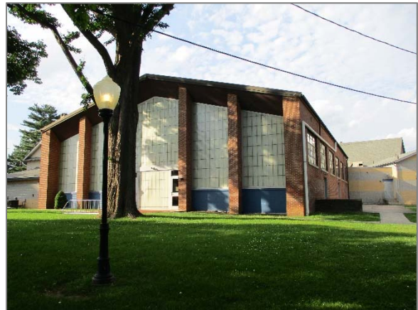
Community Center at the Fellowship House
