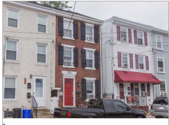
Residential dwellings along E. Elm Street
