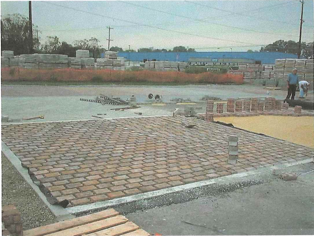
2A stone subbase Eco Paver pad
