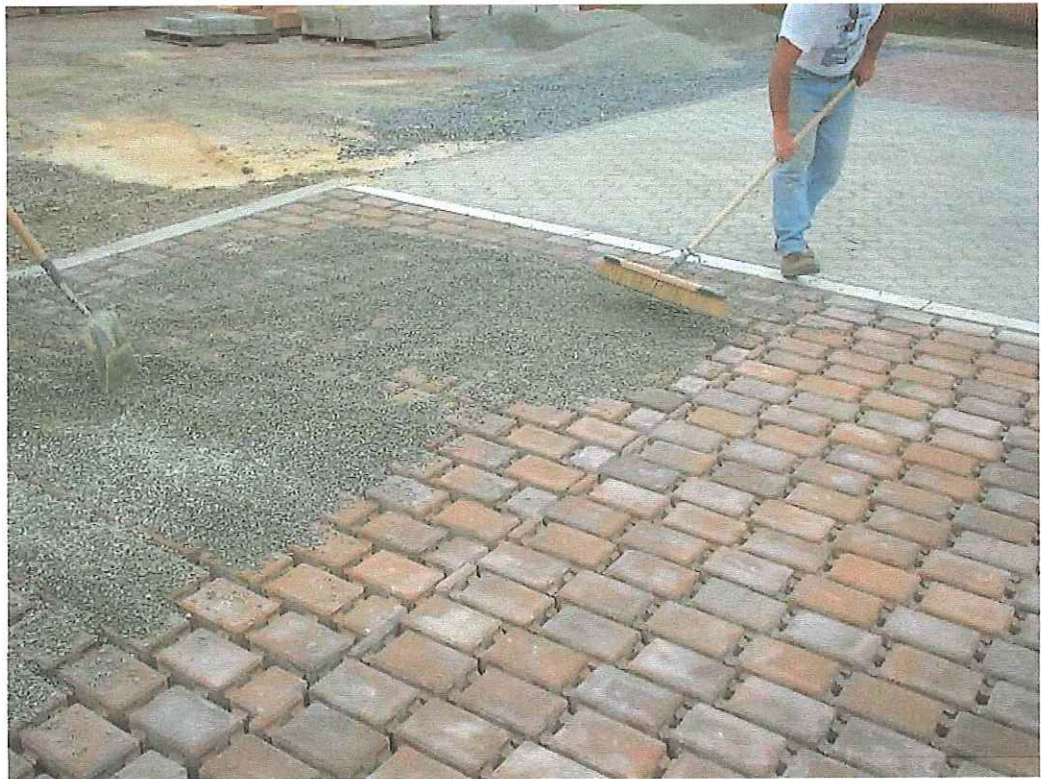
Pea gravel placement between Eco Paver units
