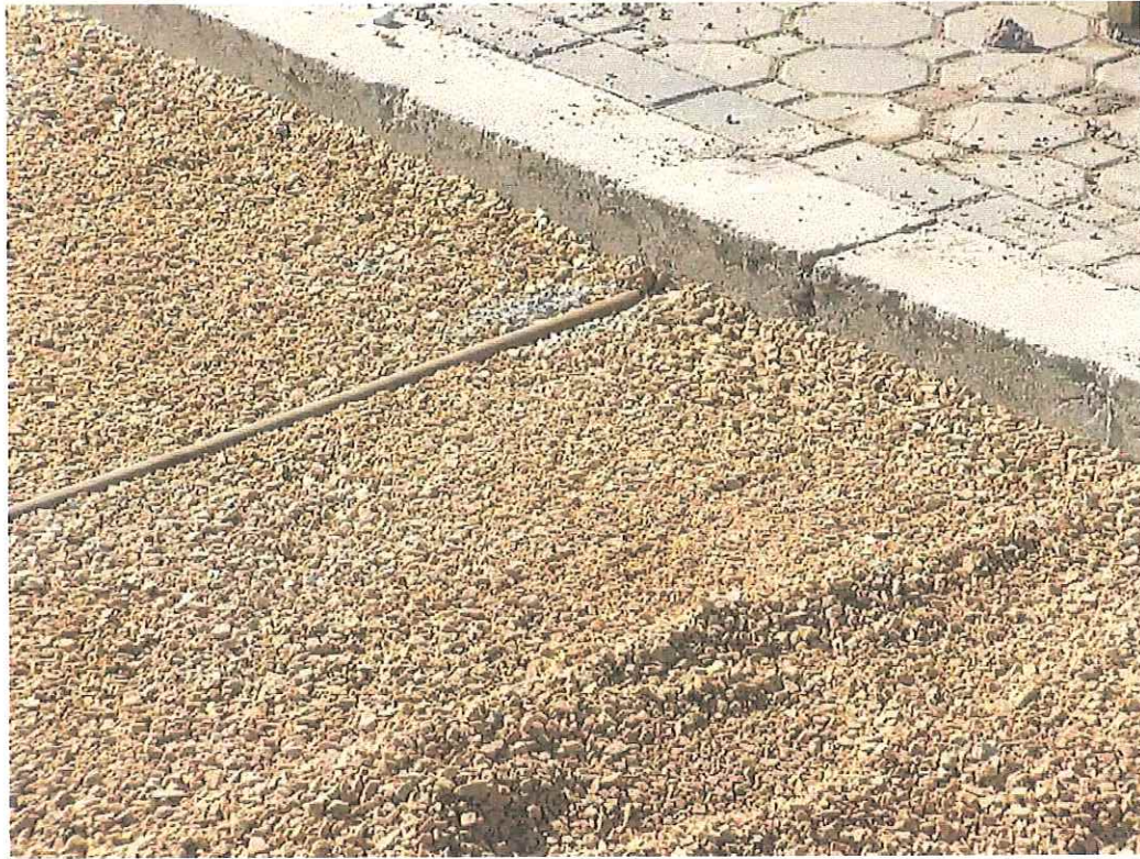
Eco Paver pea gravel leveling pad
